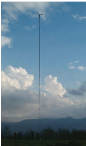
Southwest windpower H40 on an 80 foot tilt-up tower at the North Carolina small wind research and demonstration site on Beech Moutnatin, NC. Photo curtosy of NREL PIX and Appalachian State University's Dennis Scanlin.
