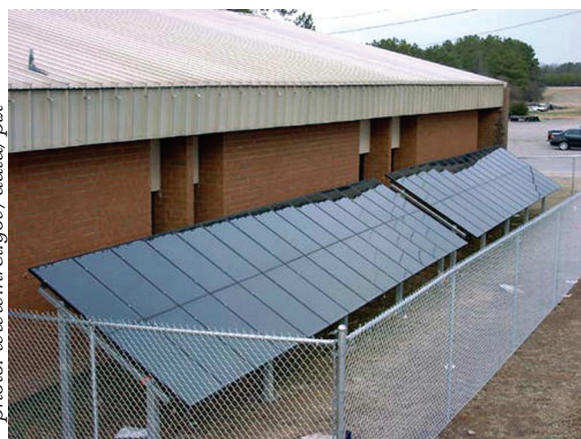
Northern Vance High School: Electric vehicle charging station, 2.6 kW dc , manufactured by BP
