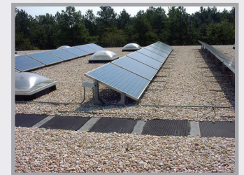
10 kW PV system installed at Intek Corporation's Aberdeen, N.C. facility Photo Source: NREL PIX
