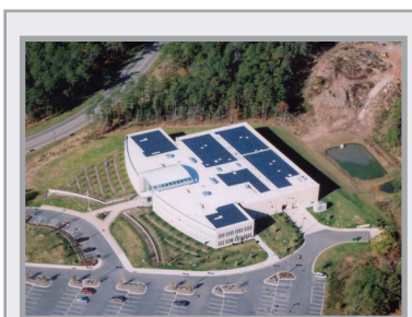
Photovoltaic system on the EPA's Research Triangle Park (RTP) facility Photo Source: NREX PIX
